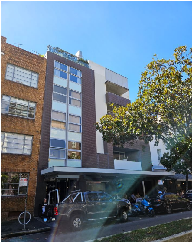
adjoining site to west - 12-16 Challis Avenue
